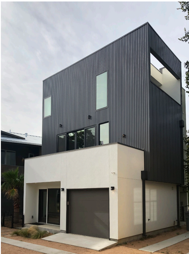
Figure 8. Infill House. Photo by author.
