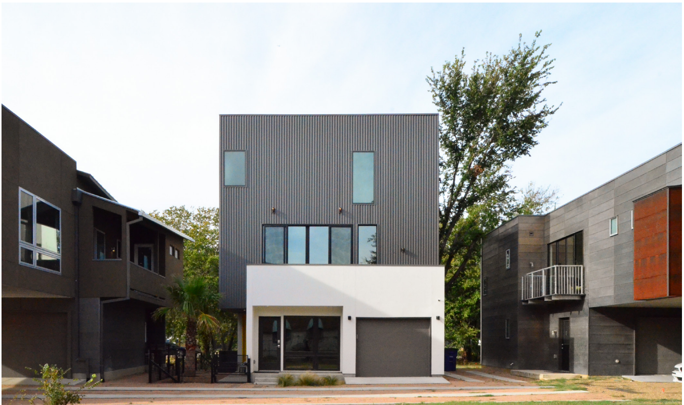
Figure 6. Infill House. Photo by the author.
